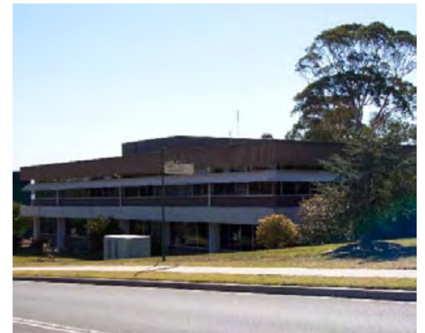
Council Administration Building near the site
